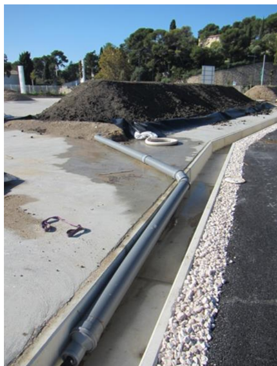
Figure 3: Pilot landform and its percolation collecting system
